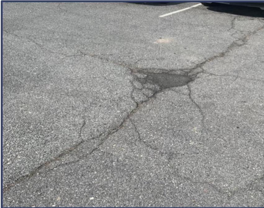
Cracks and patches in staff parking lot
